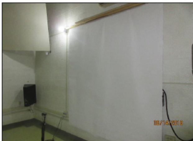
Photo No. 1 View of Installed specimen
